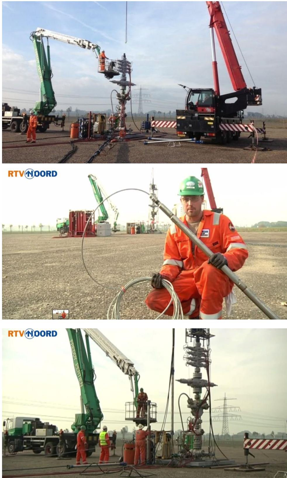
Figure 3.10 Installation of the temporary deep geophone string in well Stedum-1. .
