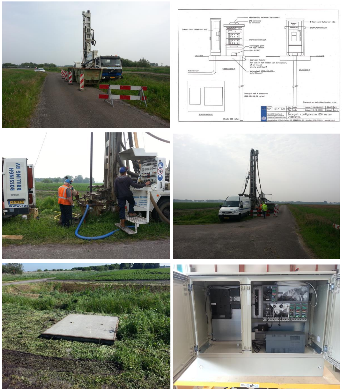
Figure 3.7 Extension of the shallow borehole geophone network.
