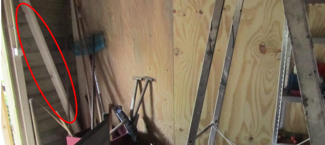
Figure I.1 Bracing in the wooden shed where BOWW is located
