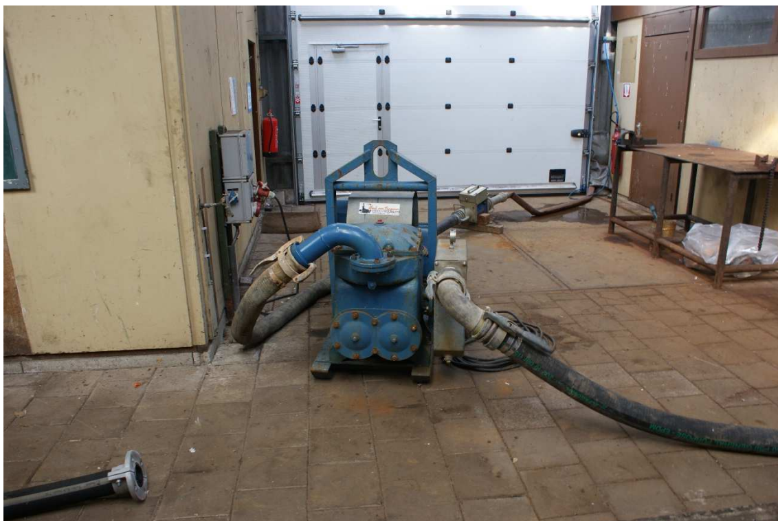
Figuur 2.5 Pomp in te slopen loods
